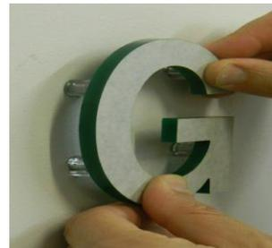
5. Fill the drill holes with a generous amount of 3M Commercial Grade Adhesive. Coat the studs with the same adhesive.
